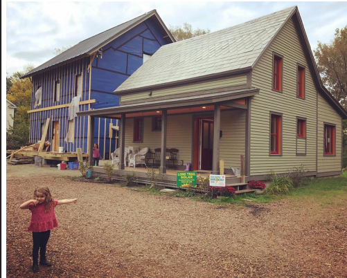
Burlington Home Energy tour attendee visiting a net zero, 19th century cottage refurbished using passive house standards.
